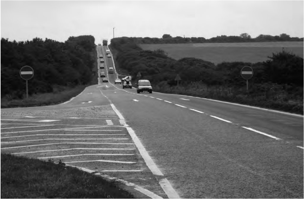
Figure 2. View from section C1 looking west with C2 to the left, N1 and N2 to the right. Photograph: Paul Chanin.
